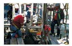
A beam-mounted milling machine was painstakingly repositioned for each sole plate. Result: validation or recalibration for all plates, well within the required tolerance.
